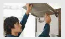
Tool-free front assembly to the lift mechanism using CLIP technology.
