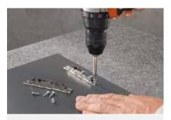
Screw on front fixing bracket in marked positions
