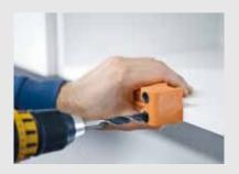
For drilling assembly, the TIP-ON unit is drilled in the centre of the cabinet base.
